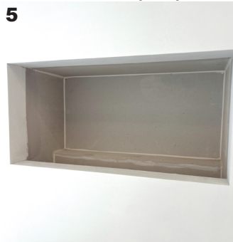
5 The fireplace wall must be hermetically sealed at the top, sides, and bottom.
