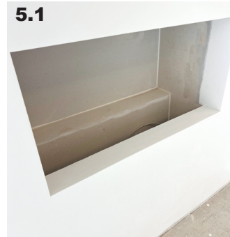
5 The fireplace wall must be hermetically sealed at the top, sides, and bottom.
