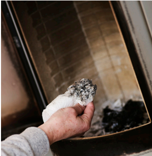
Clean the inside of the glass with a damp cloth dipped in the very fine ash inside the stove.
