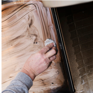
Clean the inside of the glass with a damp cloth dipped in the very fine ash inside the stove.
