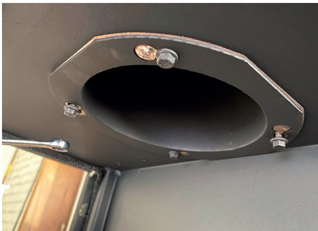
1. Loosen two of the bolts diagonally.
