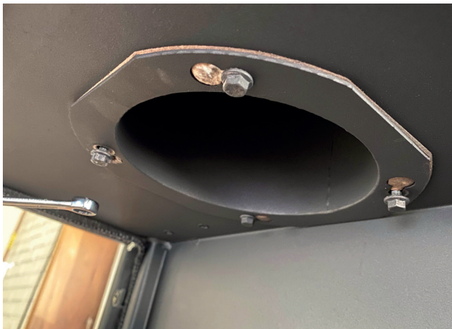
1. Loosen two of the bolts diagonally.
